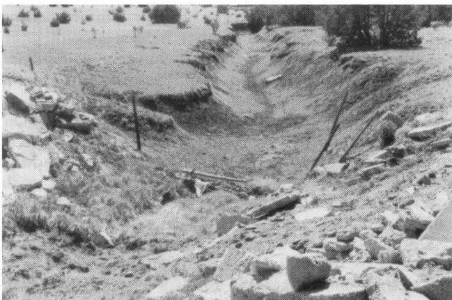
Roadside, BLM range, New Mexico. Waste concrete has been dumped along a culvert (itself quite large to accommodate runoff from damaged watersheds) to help prevent road erosion.
