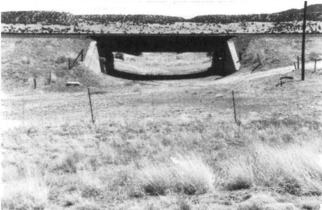
Special railroad underpasses for ranching roads and livestock movement cost railroads millions of dollars altogether. This one is not a drainage. Note the roadside fenceline contrast.
