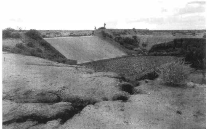
This cutbank stabilization structure on BLM range in Socorro County, New Mexico, probably cost several hundred thousand dollars. Note the size of the human figures at top-center.
