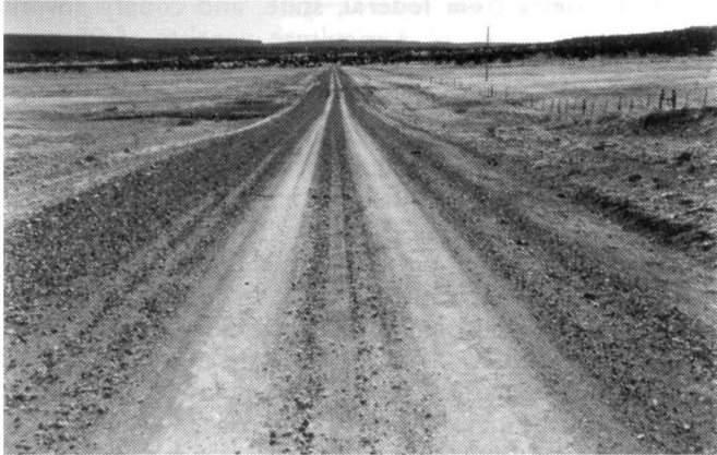
This gravel ranching road on BLM land in New Mexico is elevated, drained with ditches and culverts, reflector-marked, signed, and fenced on one side -- all at public expense.
