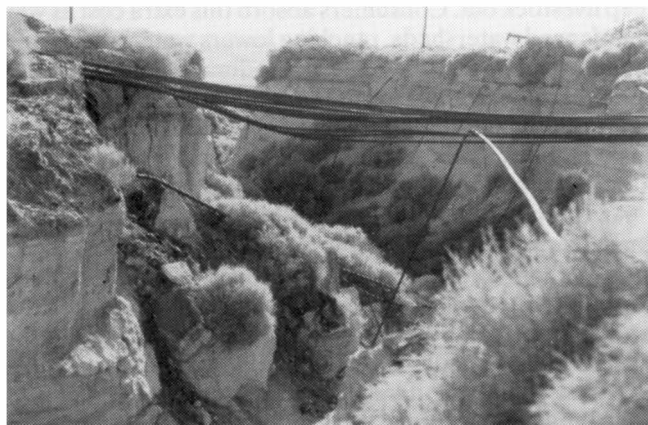
Fifty years ago these oil field pipes in California were underground. Severe downcutting, caused mostly by an overgrazed watershed, has left them useless.
